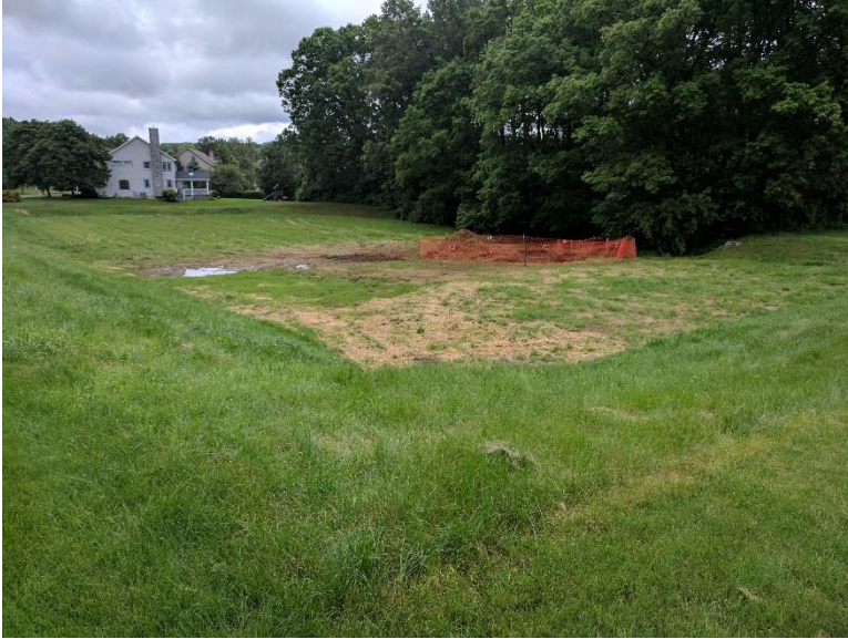
Photo 22 Additional basin modification were completed on 6/7/17
