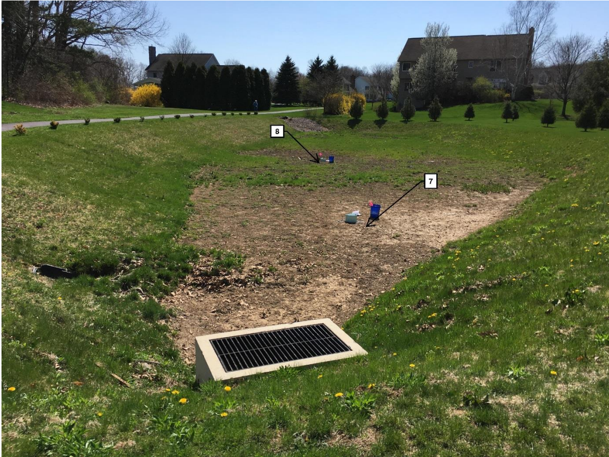
Figure 3. Test pit/infiltration test locations within the Basin 3.
